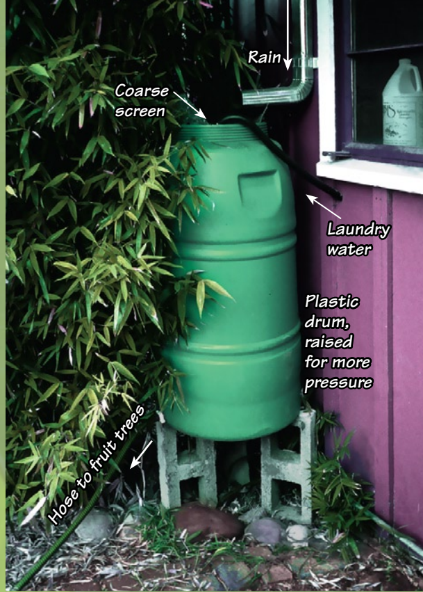
Simple Laundry Drum with Rainwater Harvesting
