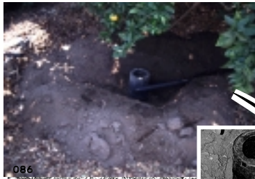
Photo 25: A sturdily made mulch basin. It is deep & wide, with thick walls. The outlet chamber in the middle is a five gallon flowerpot.
