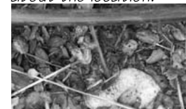
Hole drilled in tubing as emitter. Seems like cheating, it's so easy, but they're working great so far. Put them on the bottom of the line so greywater isn't geysering everywhere. A 7/32" (5.5 mm) hole is the right size to be able to plug them with drip "goof plugs" if you change your mind about the location.
