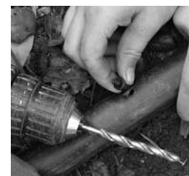
Hole drilled in tubing as emitter. Seems like cheating, it's so easy, but they're working great so far. Put them on the bottom of the line so greywater isn't geysering everywhere. A 7/32" (5.5 mm) hole is the right size to be able to plug them with drip "goof plugs" if you change your mind about the location.
