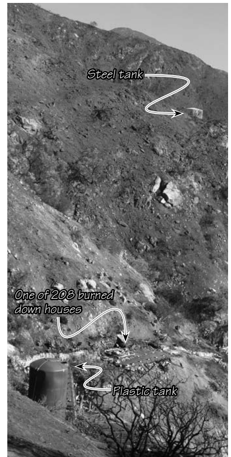
Almost all water tanks survived the 2008 Tea Fire in Santa Barbara, CA, somewhat worse for the wear, but still watertight. Several ferrocement tanks did well.
